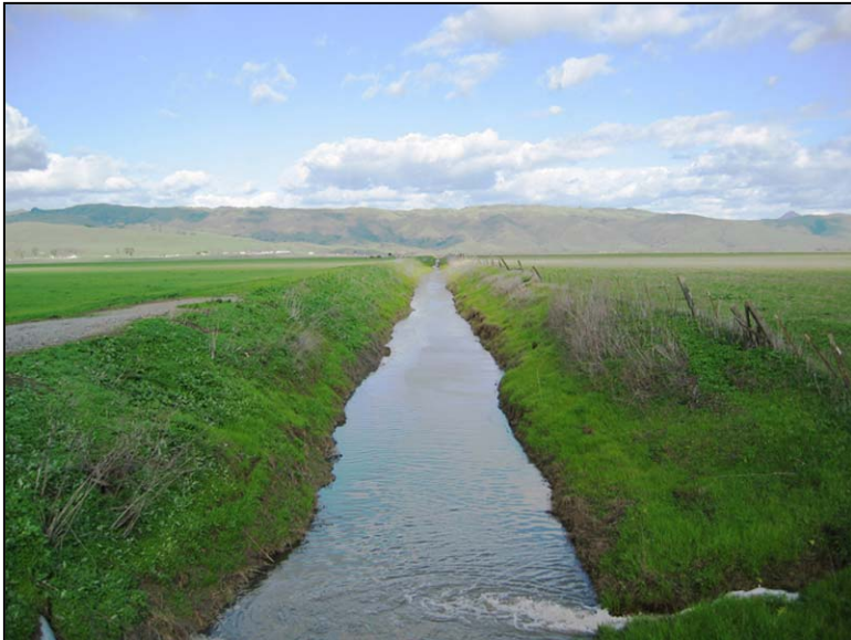
Photo 2. Millers Canal looking northeast from Frazier Lake Road
