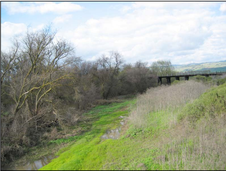
Photo 5. Pajaro River, with railroad trestle, looking north from Highway 25.
