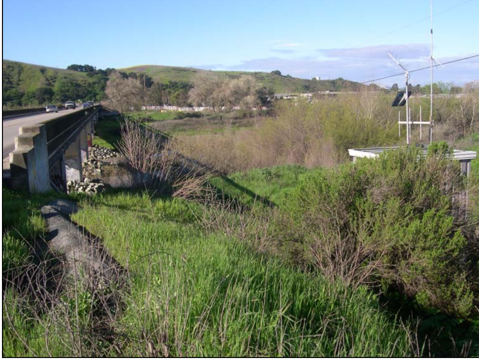
Photo 1: Looking southwest along the downstream face of the San Juan Road bridge over San Benito River. The gage house is located at right center, behind the vegetation.
