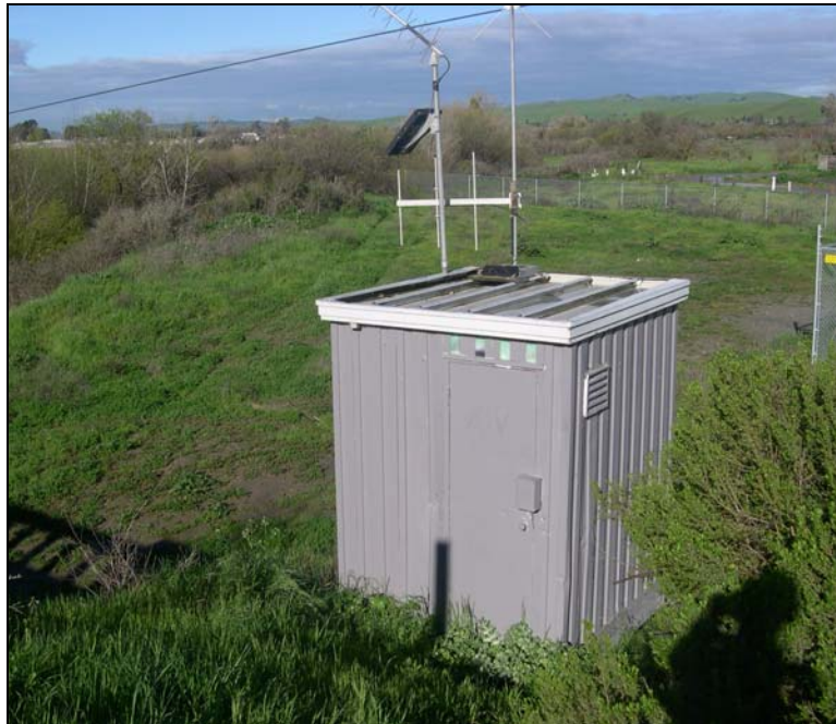
Photo 2: Gage House for USGS San Benito River at Highway 156.
