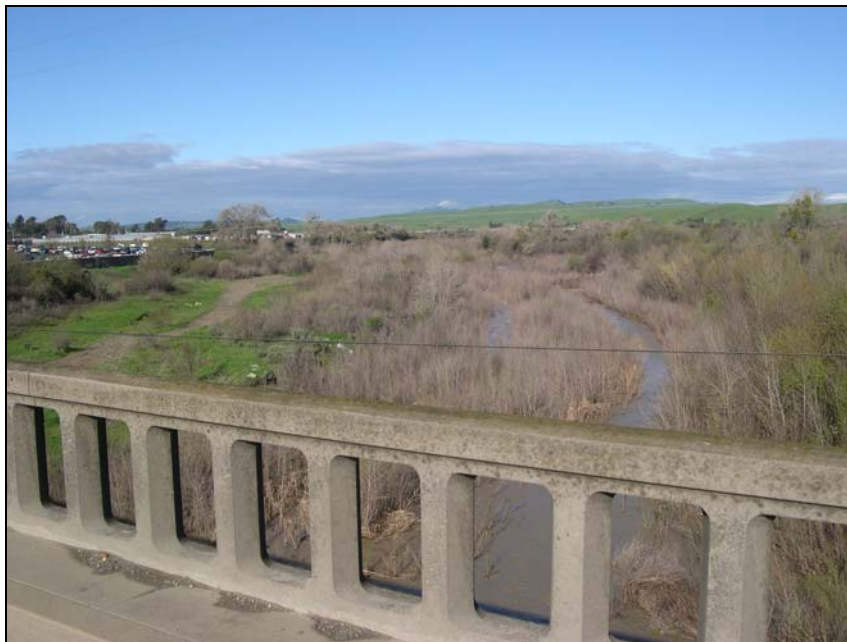
Photo 4: Looking downstream at the San Benito River from San Juan Road Bridge
