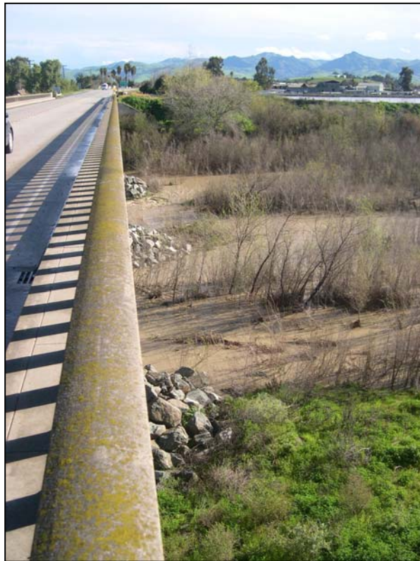
Photo 5: Looking northeast along the upstream face of the San Juan Road bridge at San Benito River.
